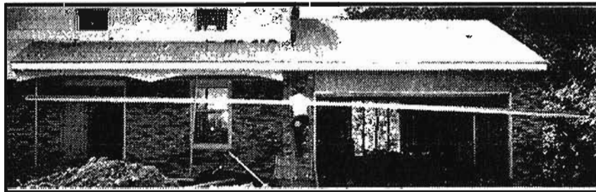
A balancing act ( a 45 ft. section of gutter)
